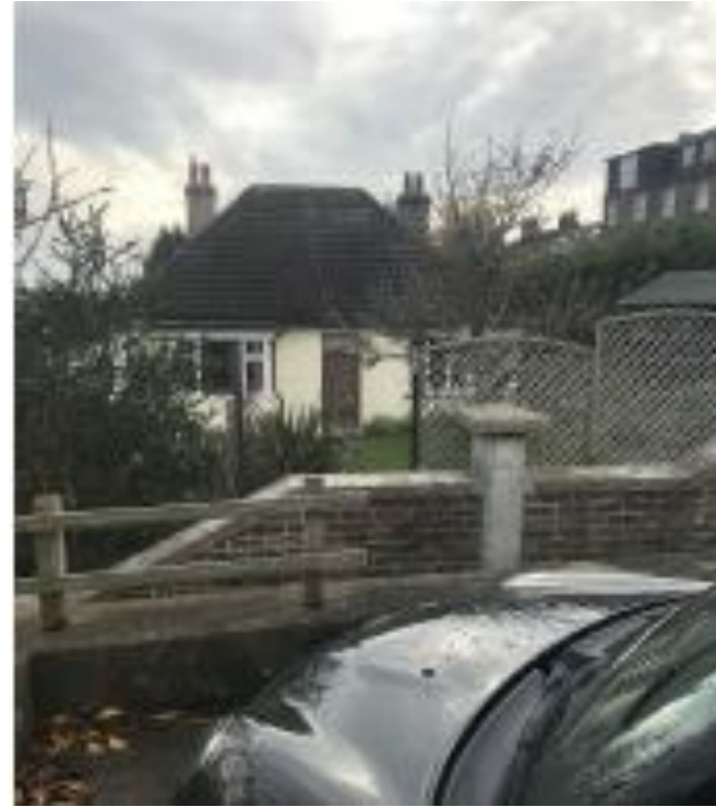
Views towards No.68A to the south
